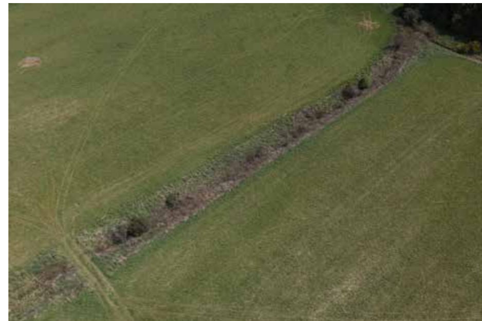
Figure 1.5 Existing drainage channel running between fields 1+2. Source: Cheal
