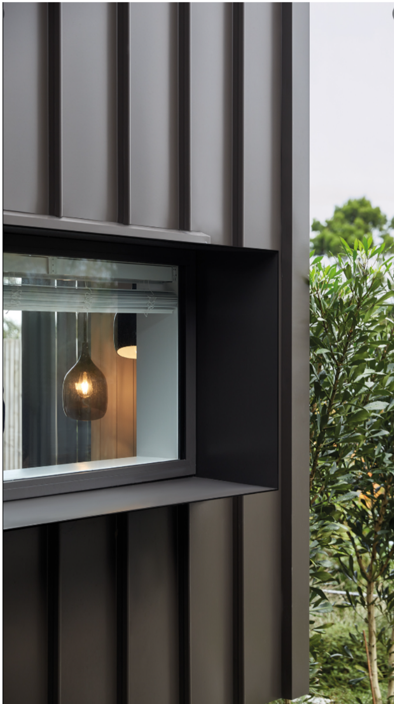
METAL CLADDING & JOINERY SURROUND
