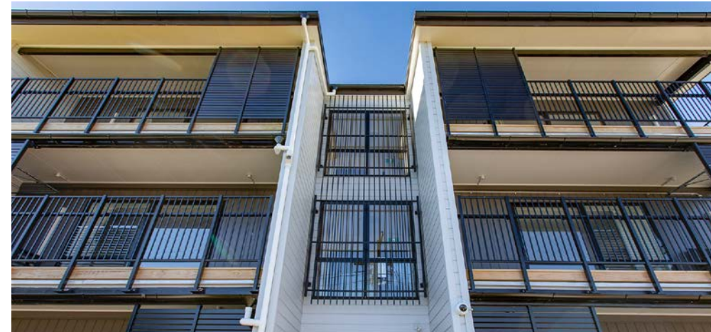
Busby Street development, Blockhouse Bay
