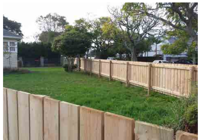
The new fence ready for the customer to return home
