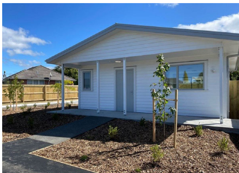
This home in Hoon Hav in Christchurch was built using the Housing Delivery System
