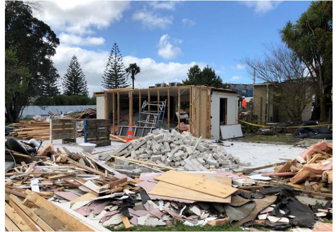
45 existing houses in an Avondale development were removed using deconstruction
