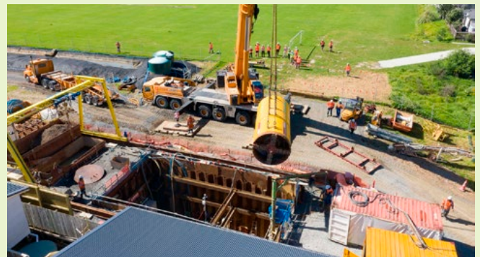
The tunnel boring machine is lowered into a seven-metre deep hole.
