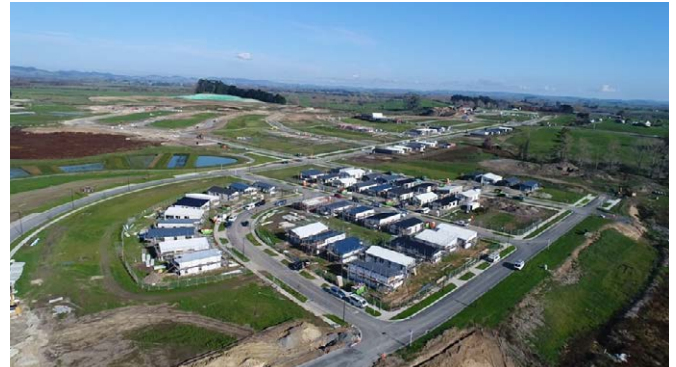
Construction is underway at the Lakeside development, Te Kauwhata.
